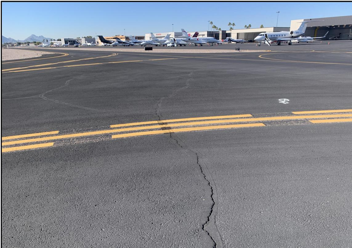
**TRANSVERSE CRACKING THROUGH EXISTING CRACK SEAL**
