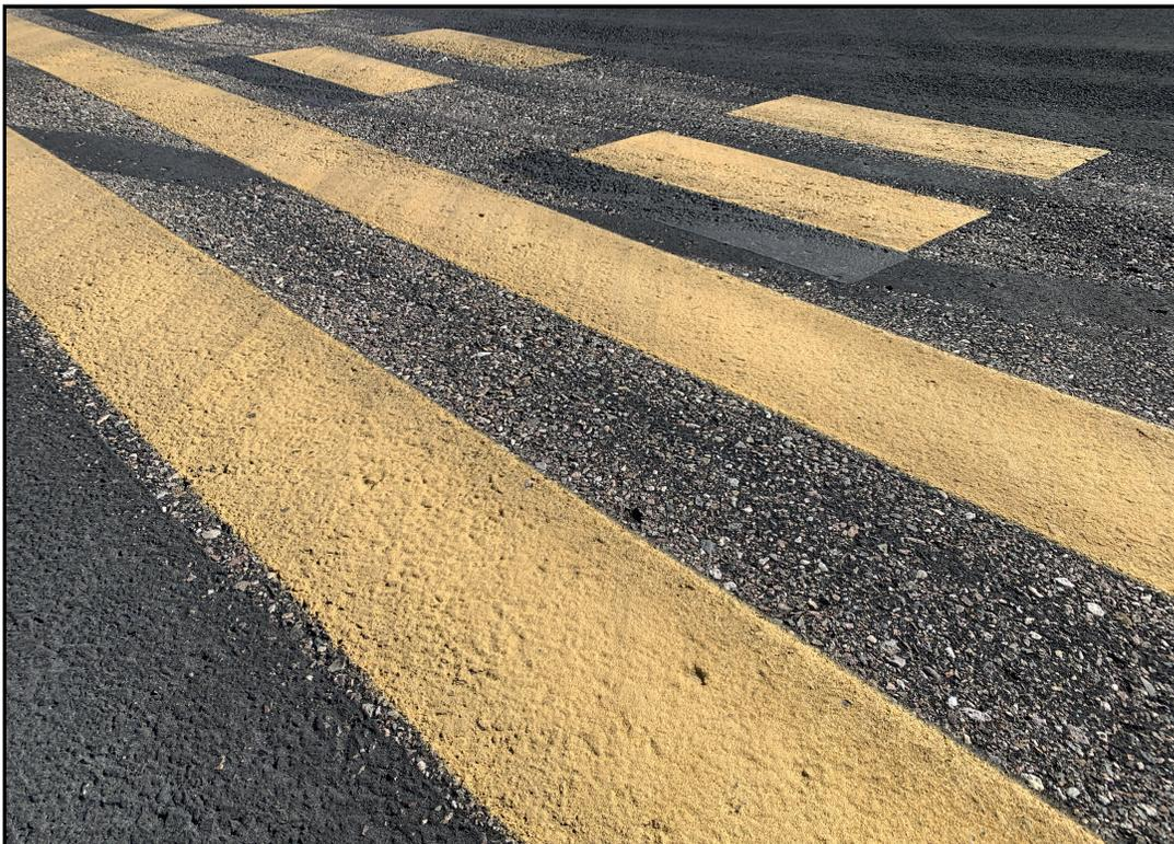
**WEATHERING OF ASPHALT PAVEMENT IN LOCATION THAT HAS NOT RECEIVED SEAL COAT SINCE BEFORE 2018**
