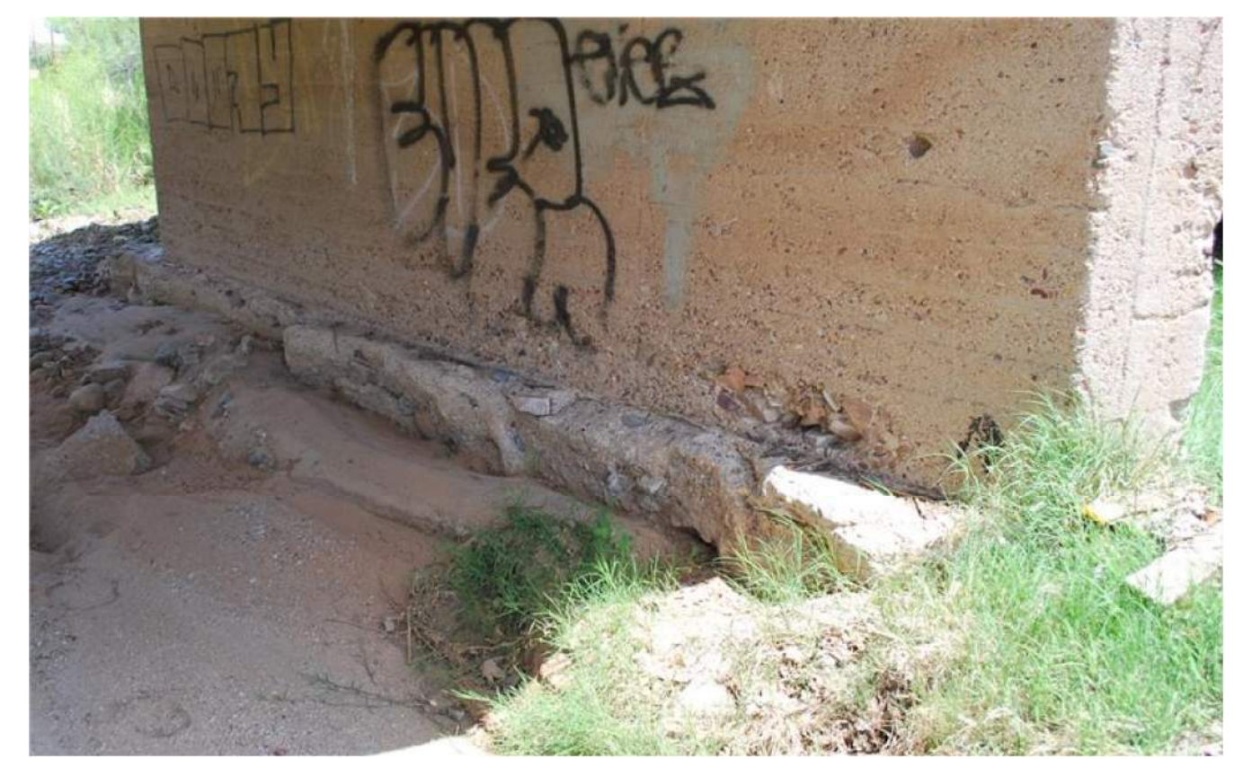
EXISTING PIER FOOTING/CAP
